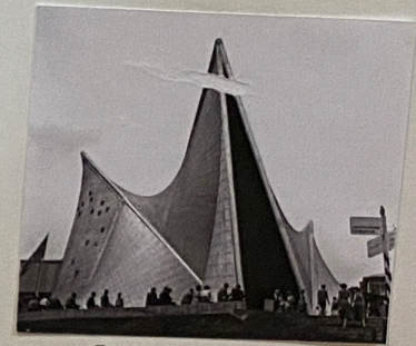
Philips pavilion Le Corbusier Belgium 1958
